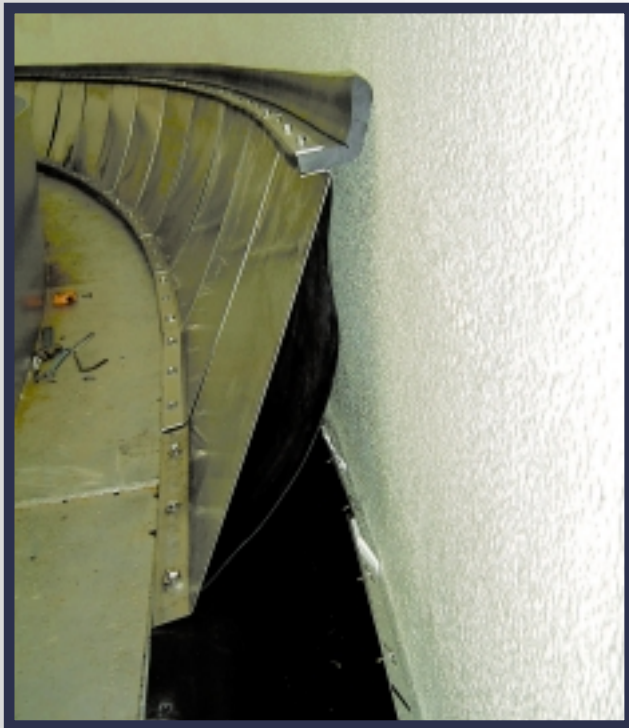
A CTS1 mechanical shoe seal fitted together with a CTS20 secondary seal represents an excellent tank seal!
