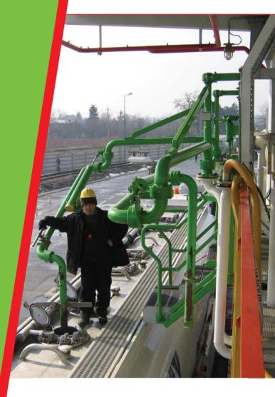
KANON top loading arms are specially designed to suit both open filling of a wide range of products across all industry sectors or closed filling of the type of highly aggressive liquids associated with the chemical and petrochemical industries.
